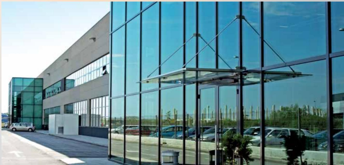
Production-business building Radin in Sv. Nedelja was built to full functionality with all construction, trade and installation works and landscaping. 13.300 m<sup>3</sup> of dam, 9.800 m<sup>3</sup> of concrete, 800 t of reinforcement, 5.4532,80 m<sup>2</sup> of prefabricated facade elements, 19.816 m<sup>2</sup> of reinforced concrete prefabricated elements (30m range construction) and 14.500 m<sup>2</sup> of traffic area.
