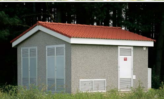
TS DTS 12 (24) - 2 x 630 (2x1000) sloping roof
