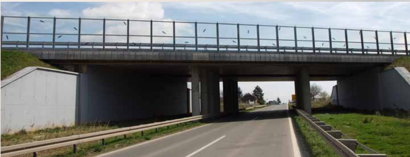
MOST na rijeci Muri, Hrvatska Bridge on river Mura, Croatia
